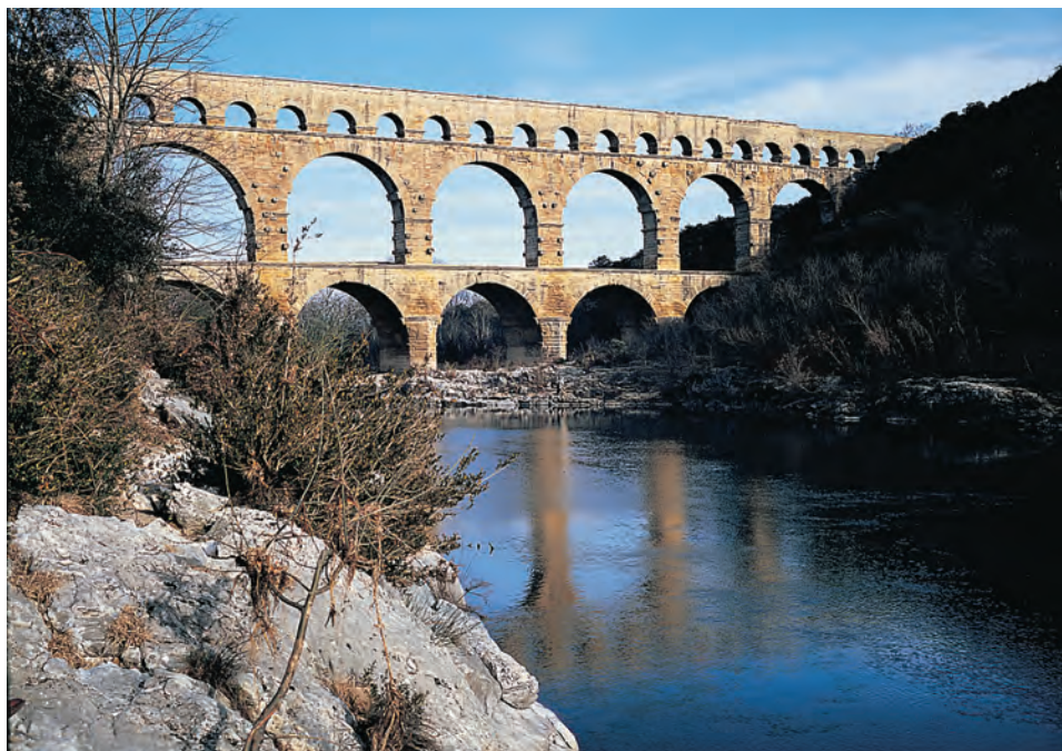
Many Roman aqueducts survive to the present day. This one carried water to the city of Nemausus in Gaul (modern Nîmes in France). The water flowed through a trough supported by the top layer of arches.
