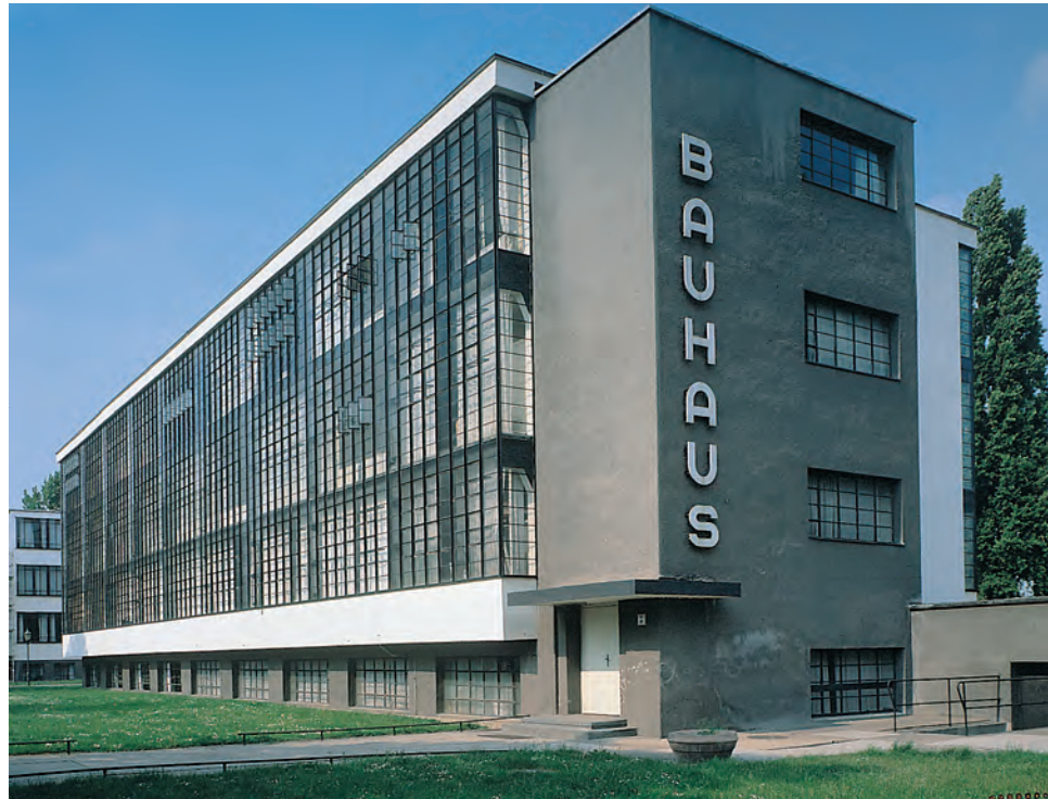
Designed by Walter Gropius in 1925, this building introduced the functional international style of architecture that dominated for the next half century.
