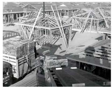
The construction of Lakewood Subdivision - note the conveyer belt to bring tiles to roof. Image courtesy of the City of Lakewood.
